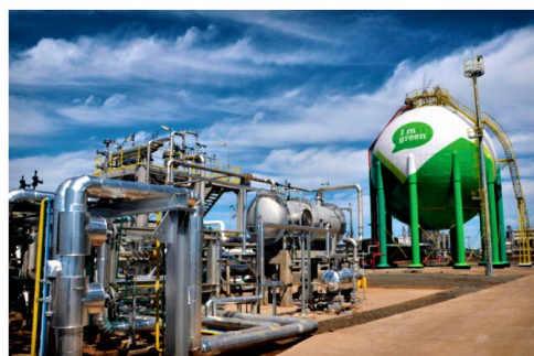
BRASKEM green ethylene plant in Triunfo (Photo: Mathias Cramer)
